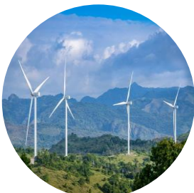
Nhon Hoi Wind Power Plant (60MW)
