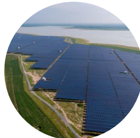
Dau Tieng Solar Power Plant (500MW)
