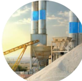
FICO Cement Factory (4.5 million tonnes/year)
